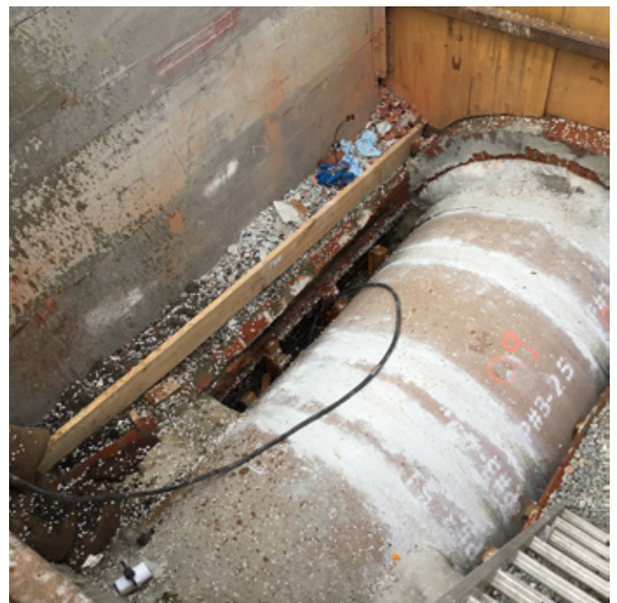
Annular grouting completed the construction process
