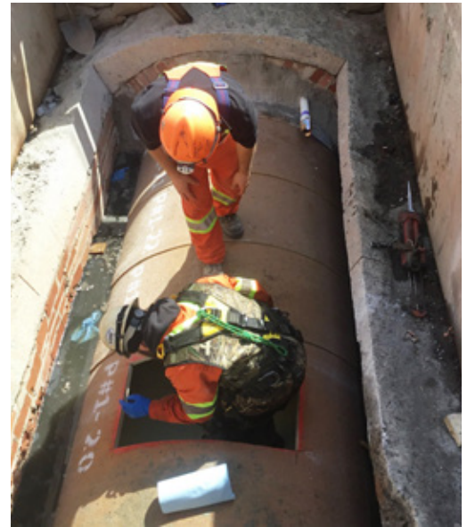
Man entry was necessary prior to grouting
