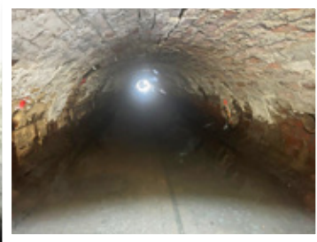
Victoria's brick sewers were built in a variety of shapes
