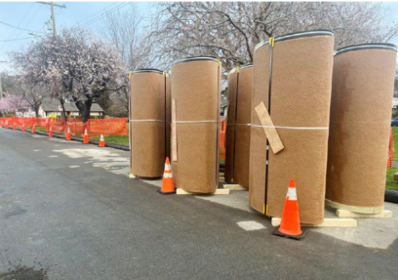
Correctly sized pipe segments were delivered to the site from Dubai
