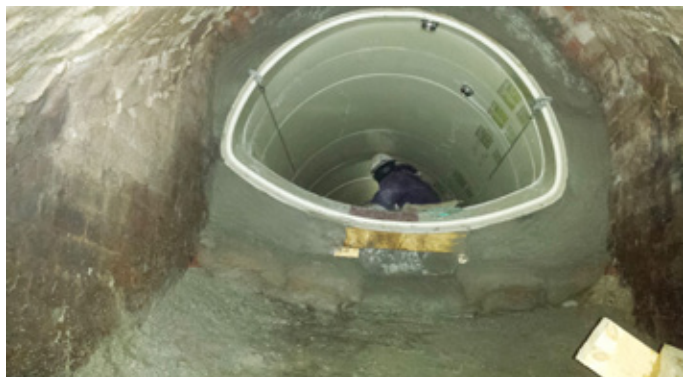
There is growing experience with using GRP liners for storm sewer applications, with an ability to be installed through major vertical and horizontal bends in the host pipe
