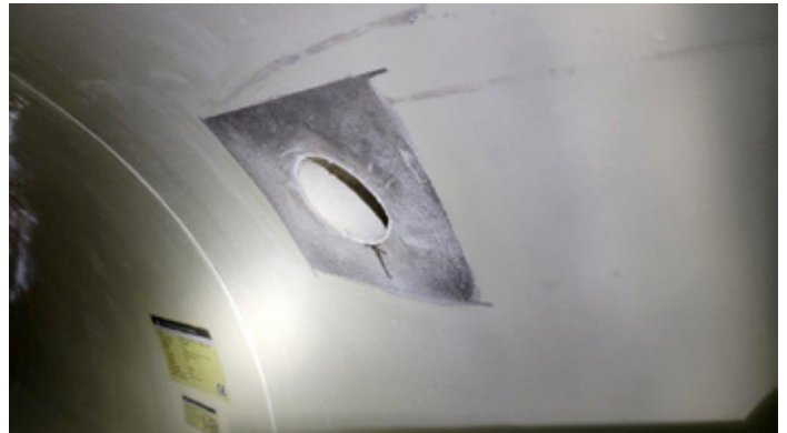
Laterals were located and cut
