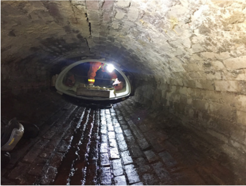
GRP liners conform to the unique shape of the existing pipe
