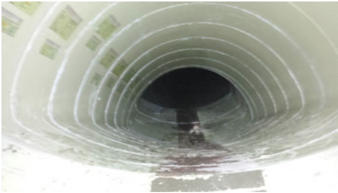
Intent of the sliplining program is a fully structural rehabilitation
