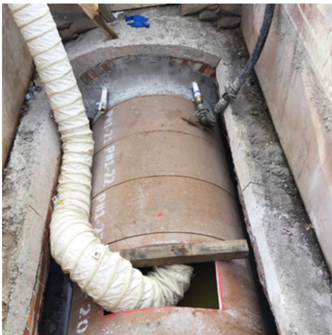
Annular grouting completed the construction process
