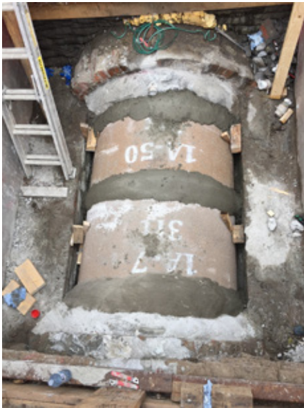
Each seam had internal gasket and external seal
